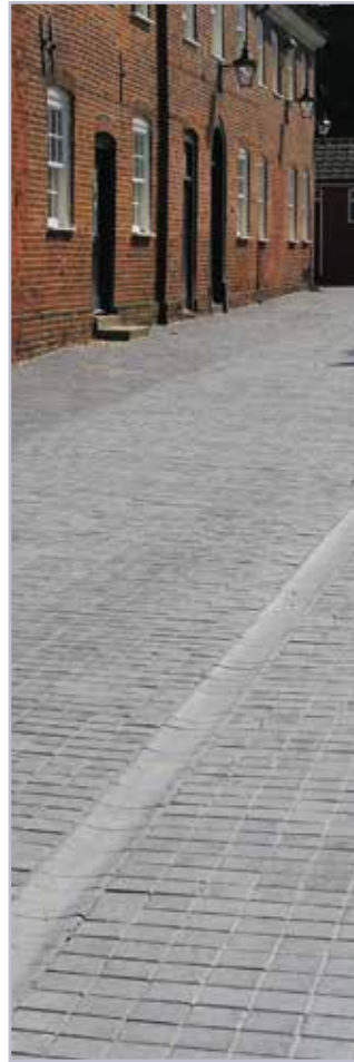
Ketley drainage channels with Ketley 2 panel pavers.
