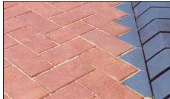
Blue standard kerbs and small triangle starter units with red pavers laid in 45° herringbone bond.
