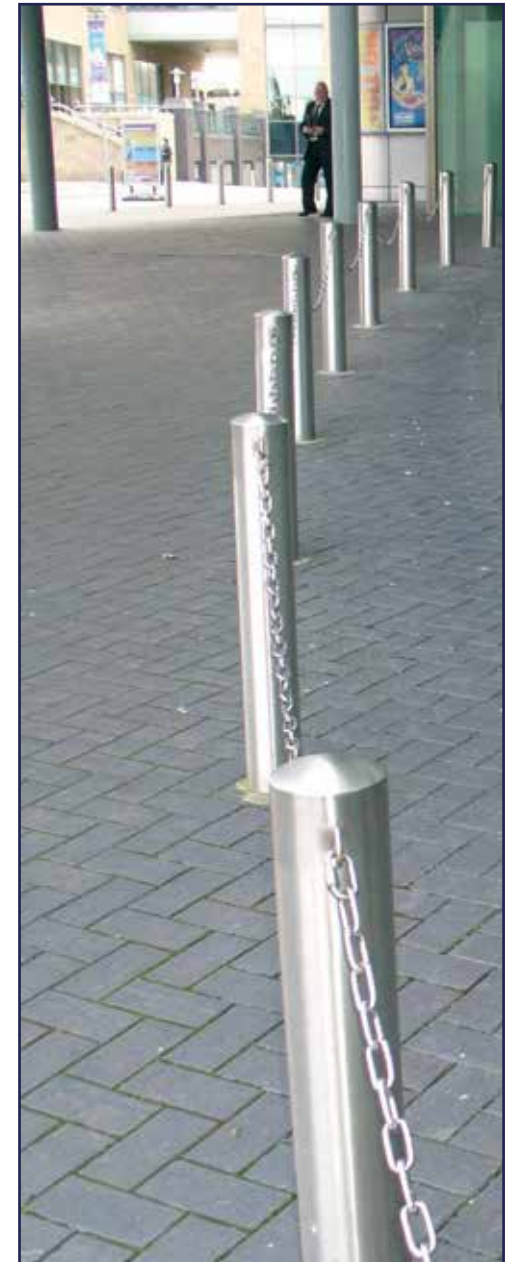
Blue plain chamfered pavers laid in herringbone bond at the Lowry Centre, Manchester.
