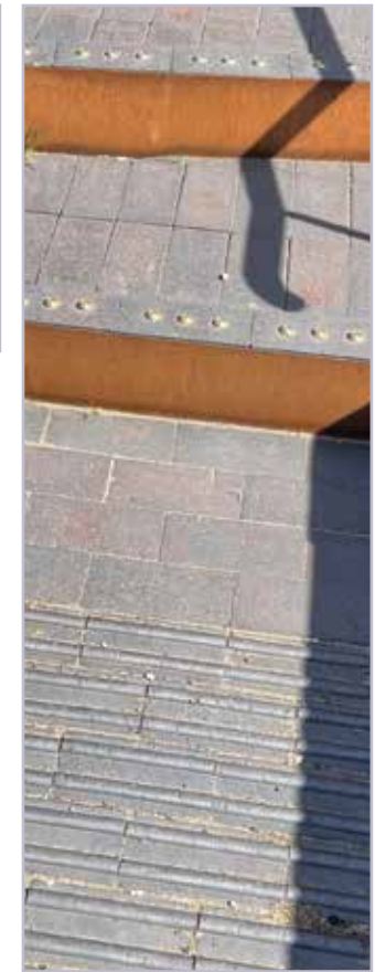
Ribbed/corduroy pavers mark the limit of the steps outside the Manchester Jewish Museum.
