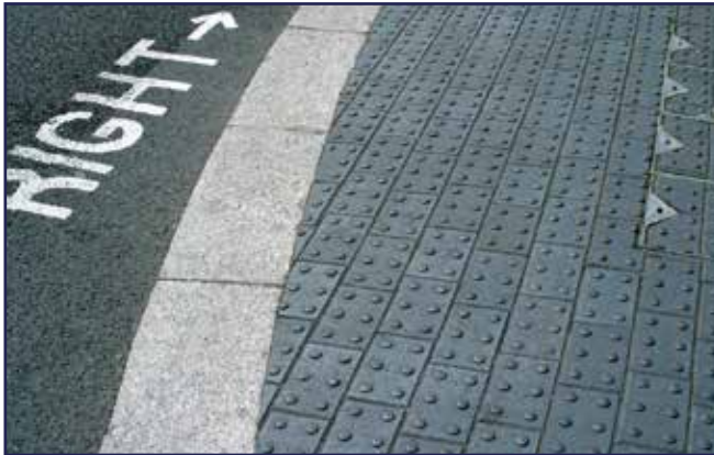
Blue tactile blister pavers in Hammersmith, London.
