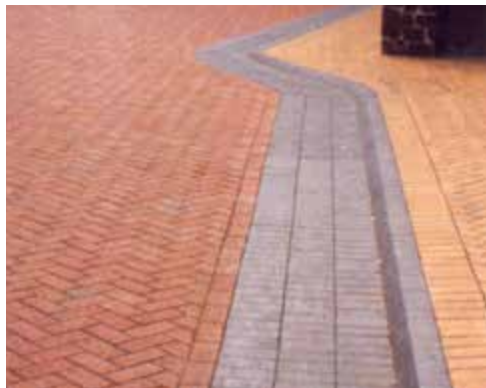
Blue Chamfered Pavers and Kerb Units - Wellingborough.
