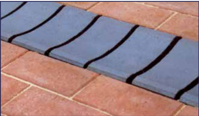
Blue drainage units with red pavers laid running bond.
