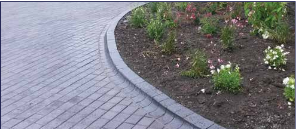
Ketley blue boot kerbs with Ketley 2 panel pavers.
