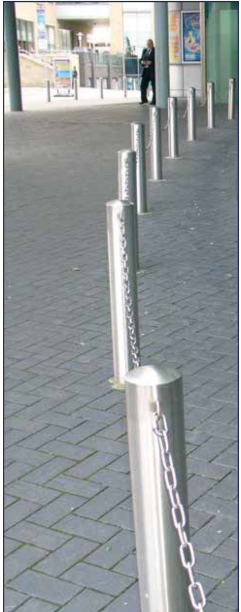
Blue Plain Chamfered Pavers laid in herringbone bond at the Lowry Centre, Manchester.
