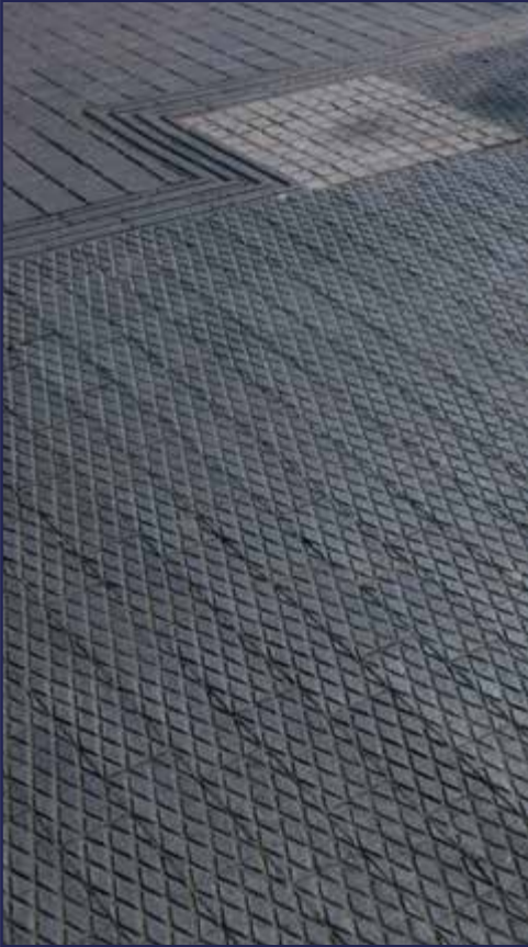
Blue Diamond Chequer Pavers laid in \frac{1}{3} running bond with Blue Ribbed Pavers and Blue 2 Panel Pavers at Camden Lock, London.
