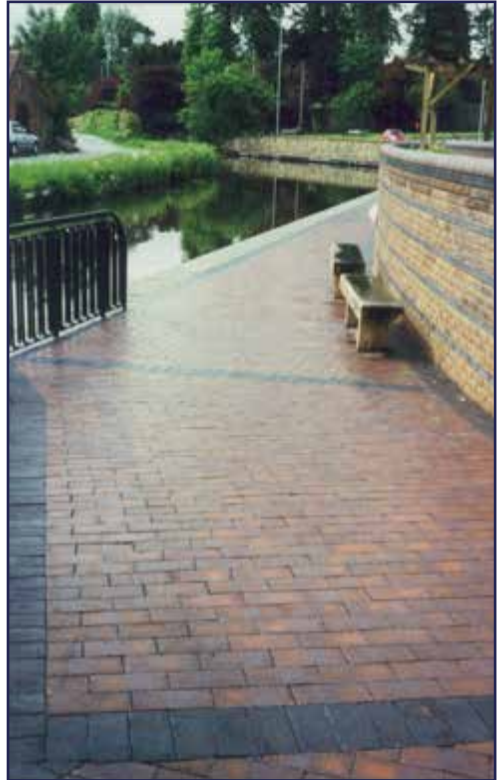
Brown Brindle Square Edged Pavers in running bond with plain Blue Square Edged Pavers at Canalside, Welshpool.
