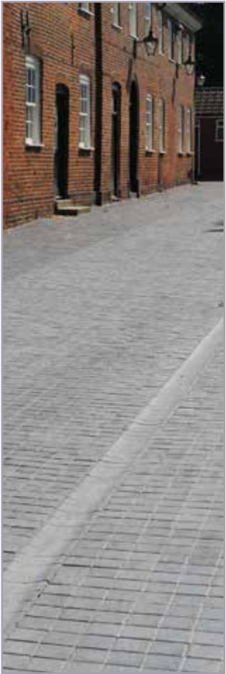
Ketley drainage channels with Ketley 2 panel pavers.
