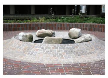
landscape features were carefully detailed to meet listing criteria, reduce dead loads on the slab and ensure longevity of replacement elements.
